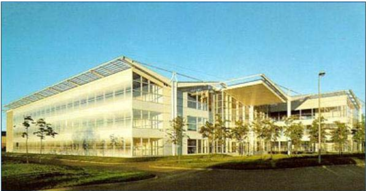
Building B3 in an English business park, built by Foster & Associates reflects a freedom of configuration and orientation allowing greater openness towards the outside world. The entry is located on the north side with its many windows, while the windowless service areas are situated on the southside. Offices thus open towards the east and west: their frosted white windows filter solar gains and diffuse the light. Atria running the length of the building connect the three units and allow natural light to reach the structure's centre.
